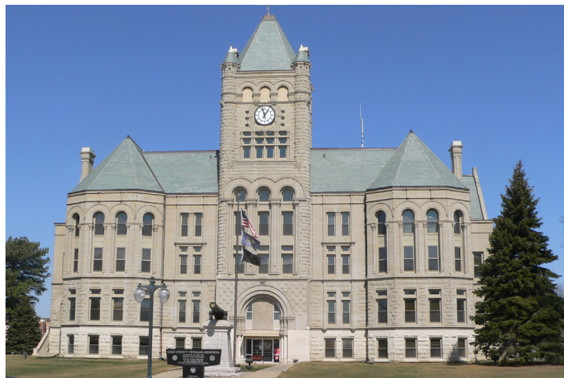
Gage County, Nebraska Courthouse. Source: Wikimedia Commons
